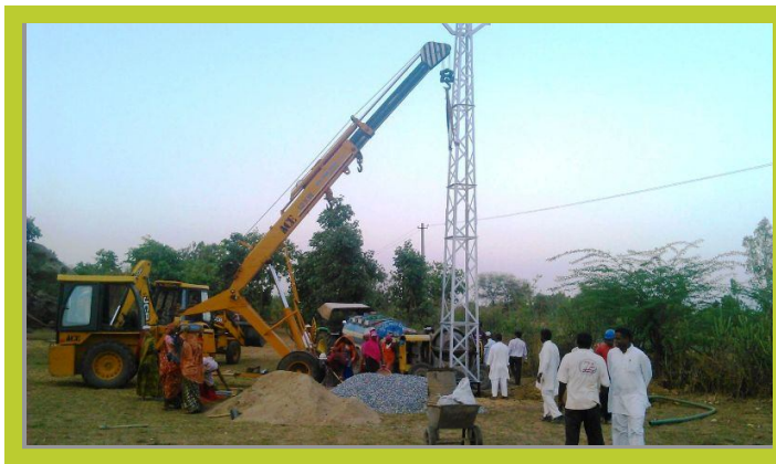
Erection of the first lattice tower; in total 24 towers were installed for 11 kV transmission lines from solar plant to Shantivan campus.
