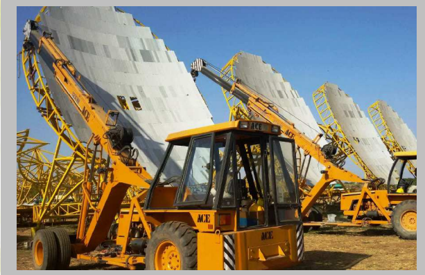
Erection of solar reflectors
