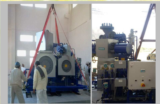
Installation and alignment of the turbine and generator
